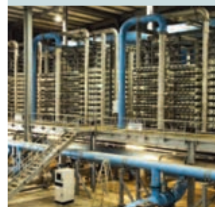
Desalination plants typically use austenitic and duplex stainless steels
